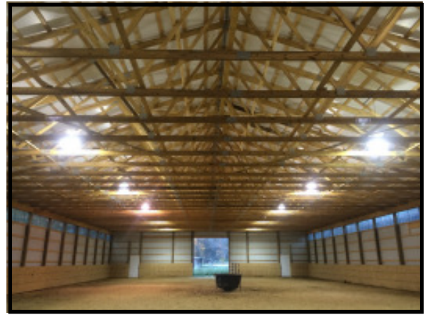
The beautiful new arena lights were installed thanks to volunteer electrician, Bentley Hudson.
